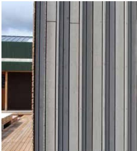
screws, which don't require pre-drilling, together with KompeFix® compensation strips to create a ventilation gap. One third of the boards benefit from the fixing-free look provided by secret-fix option FassadenClip®, with both of these fixing solutions improving ventilation and thereby enhancing the durability and stability of the timber.
