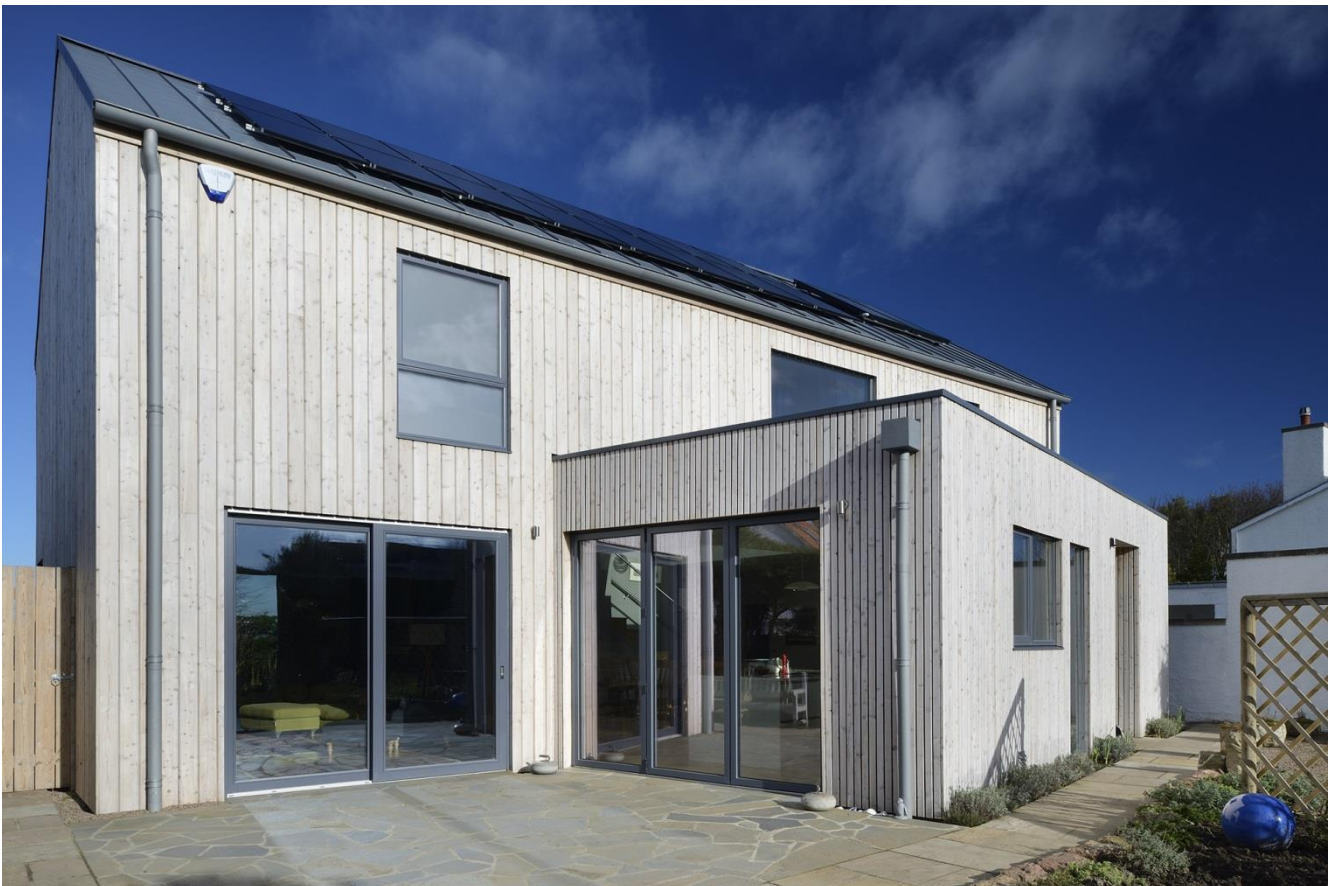
Scotlarch® with SiOO:X in East Lothian after one year's weathering.
