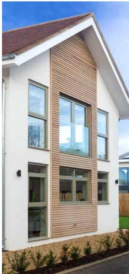
Russwood Siberian Larch SILA A/B® was the product of choice, laid in 70mm width rainscreen profile. SiOO:X treatment retains the natural beauty of the timber but allows for uniform weathering, whilst secret fixings of FassadenClip® and L-GoFix® A2 screws provide a clean, contemporary finish.
